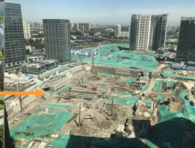
Actual site: Broke ground for the office/retail land site
